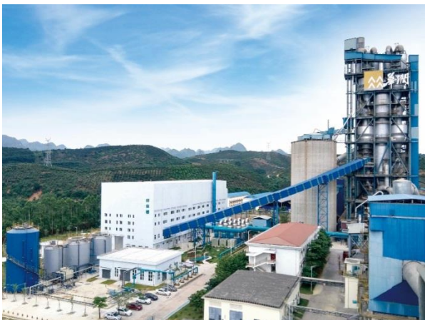
The municipal waste co-processing project in Tianyang, Guangxi
