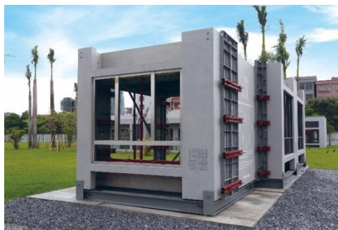
Prefabricated Construction Module
