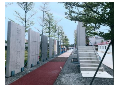
Precast Concrete Components
