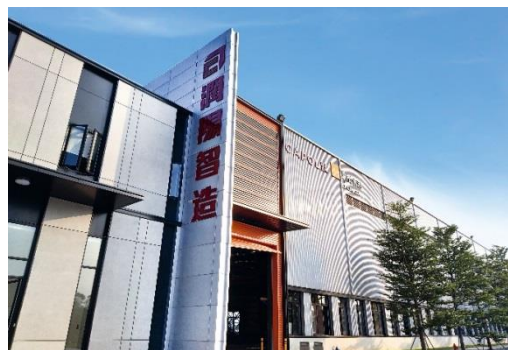
Precast Concrete Production Plant in Dongguan, Guangdong
