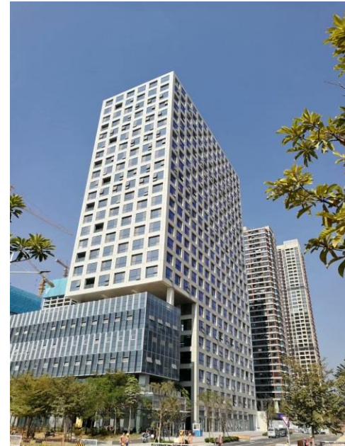
Prefabricated Building in Shenzhen: Shenzhen Vanke Yuncheng
