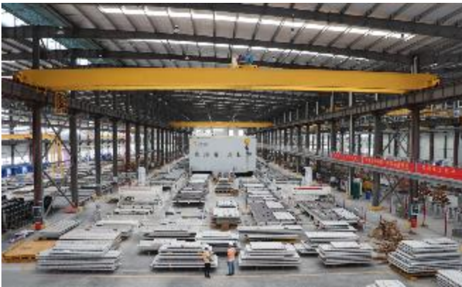
Precast Concrete Production Plant in Guigang, Guangxi
