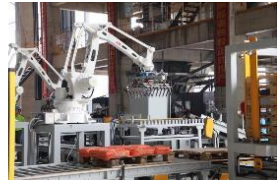
Tile Adhesive Production Line in Fengkai, Guangdong
