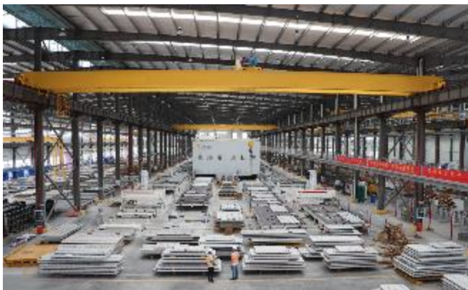
Precast Concrete Production Plant in Guigang, Guangxi
