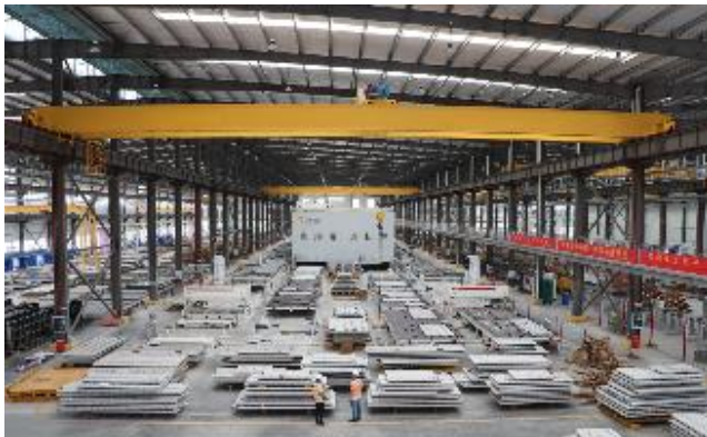
Precast Concrete Production Plant in Guigang, Guangxi
