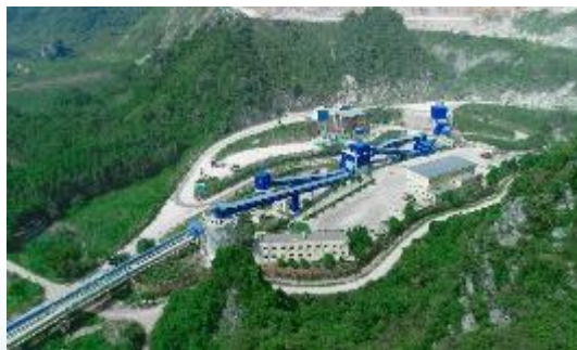
Aggregate Production Line in Nanning, Guangxi
