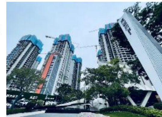
China Resources Wanyue Mansion at Pingshan, Shenzhen, Guangdong
