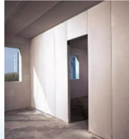
Interior Wall Panel
