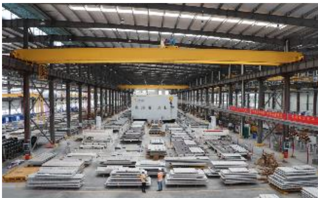
Precast Concrete Production Plant in Guigang, Guangxi
