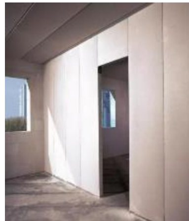
Interior Wall Panel
