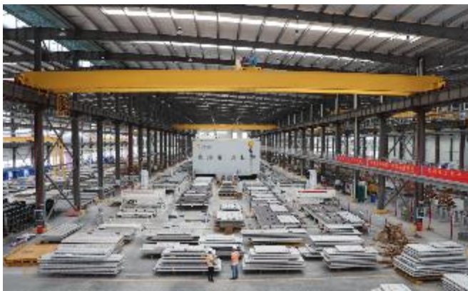
Precast Concrete Production Plant in Guigang, Guangxi
