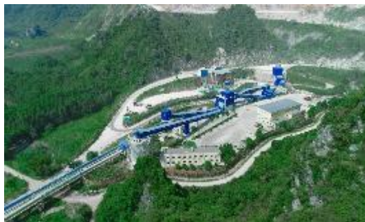
Aggregate Production Line in Nanning, Guangxi
