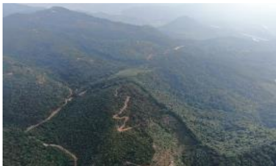
Aggregate Mine in Fengkai, Guangdong
