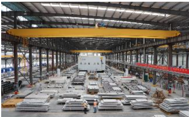
Precast Concrete Production Plant in Guigang, Guangxi
